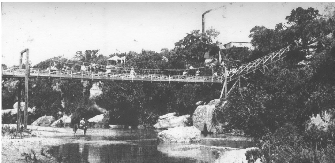
Suspension footbridge over the South San Gabriel River in Georgetown. The Chautauqua grounds are on top of the bluff on the right.
